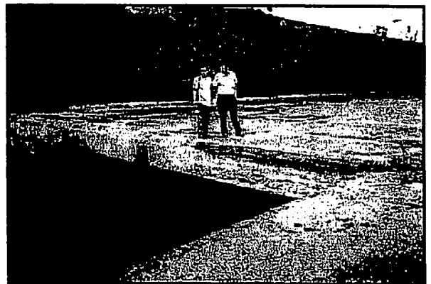
Existing Ro-Ro ramp at end side of Old Quay. Some timber waling are missing.
