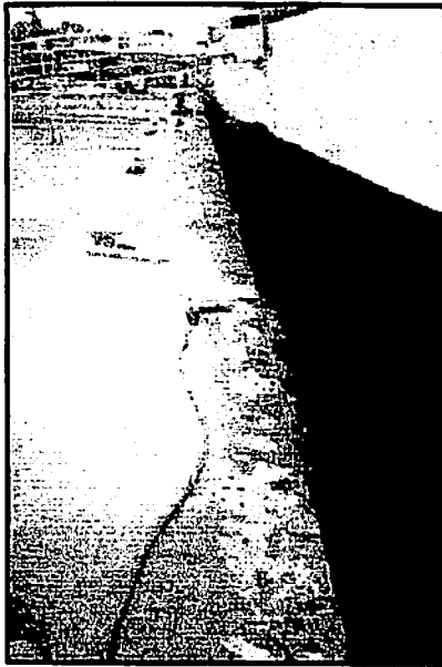
Concrete curb or cap edge eventually chipped-off to deck level.
